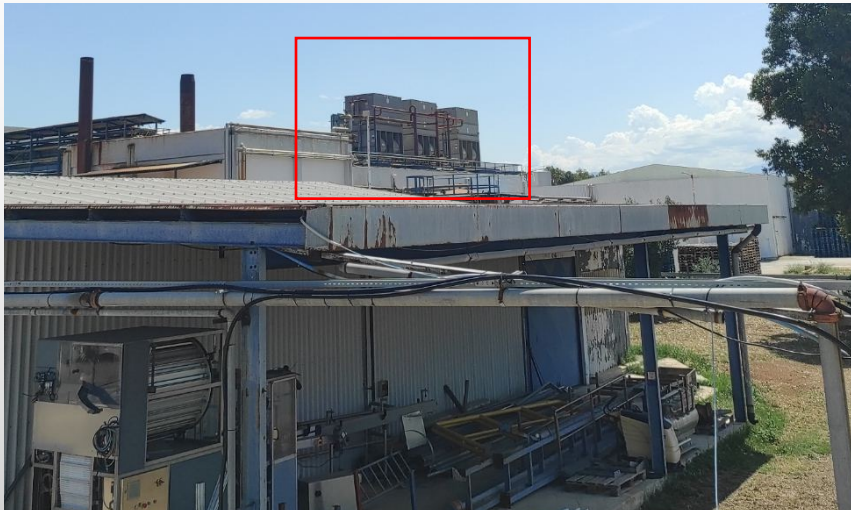
FCH – Cooling towers
