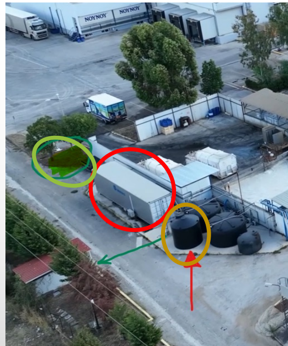
Side view of the installation area
